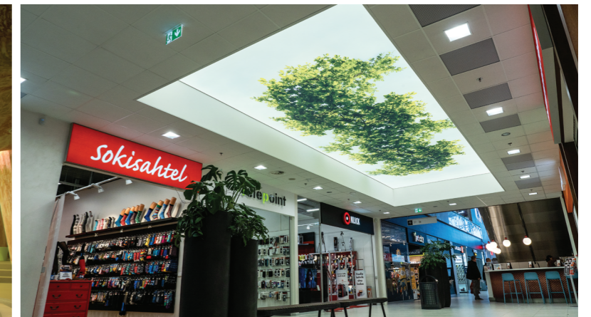
Eesden Shopping Mall Estonia / Tartu Installer: Vecta Design
